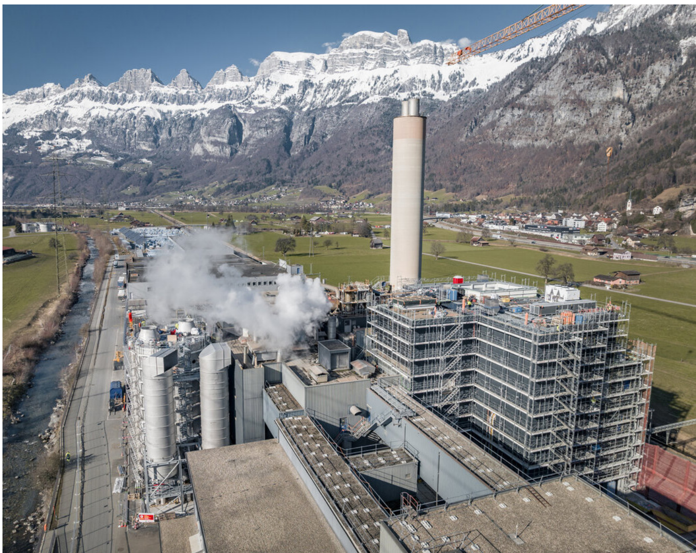
29: Flumroc, Flums, 2022 Source: Flumroc
