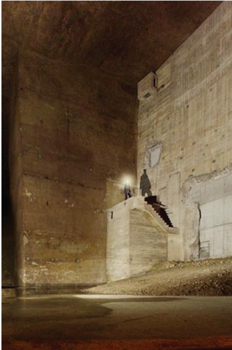
Inside the dismantled facility. The concrete foundations of the steel tanks are still visible in the front. The old quarry entrance is visible to the right (vimudeap.info)
