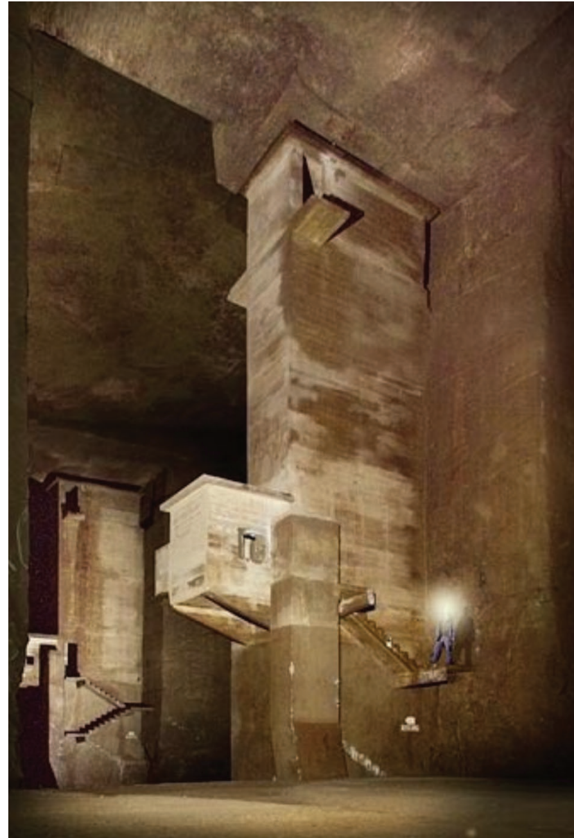
Concrete staircases were built to reach the top of the steel tanks. (vimudeap.info)
