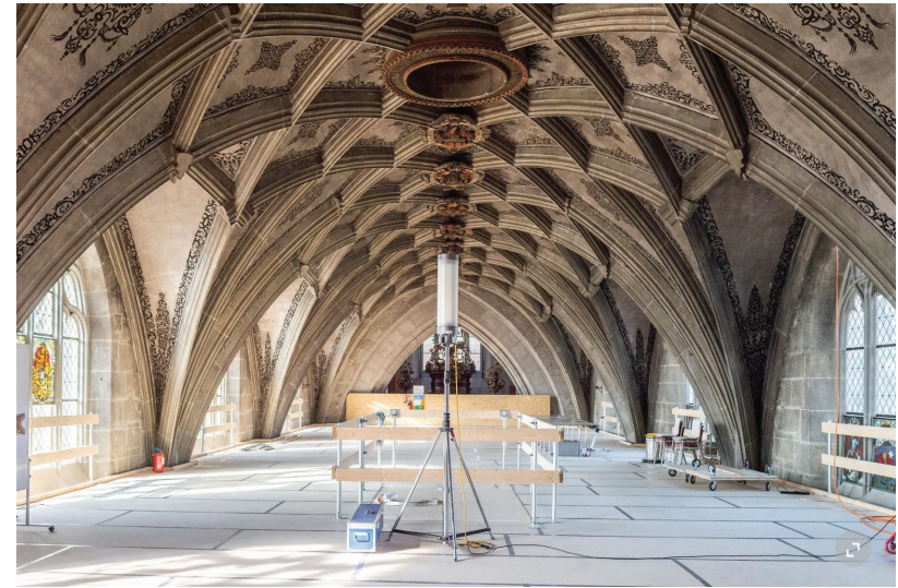
Temporary working platform and office for restoration on the vaults (bernermuensterstiftung.ch)
