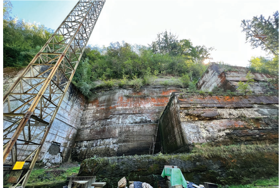
Platforms and crane
