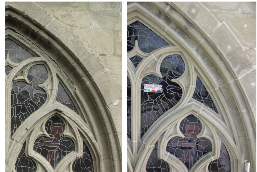
Repairing a weathered window frame on site with mortar (bernermuensterstiftung.ch)
